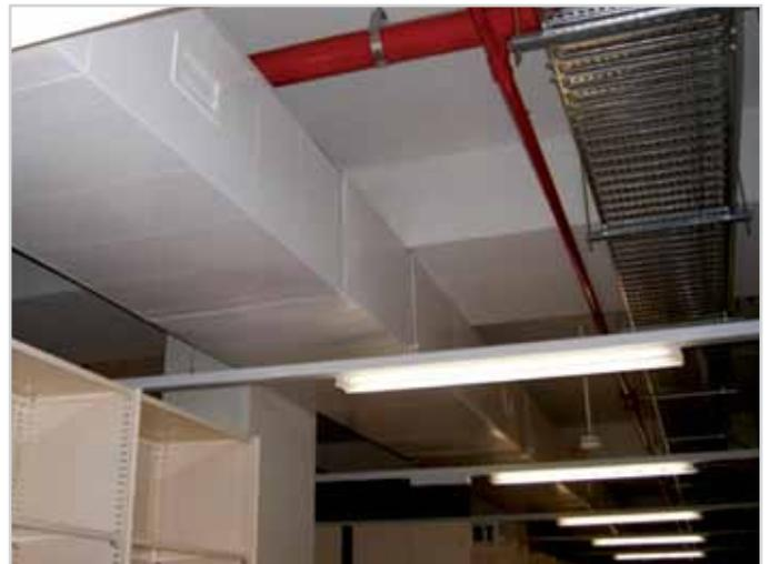
*Services resolved: as built piping and ducting which were coordinated through the 4D model*
